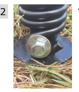
Using the wrench and ratchet, attach the spring to the stem of the ground spike with the included spring kit.
