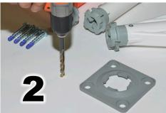
• Using a 3/8" masonry bit, drill 3" in depth
