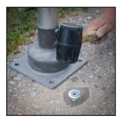
USING A RUBBER MALLET, TAP BOLTS INTO THE HOLES
