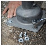
USING A 9/16" RATCHET, TIGHTEN BOLTS
