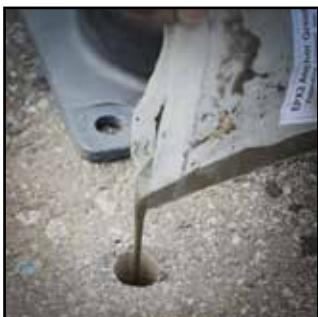
POUR MIXTURE INTO THE 4 HOLES (ONE BAG PER TWO HOLES)
