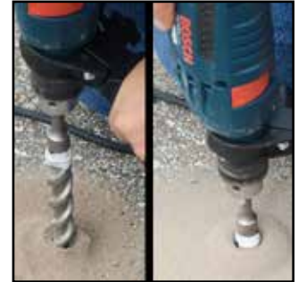
DRILL 4 HOLES 7/8" DIAMETER 6" DEEP
