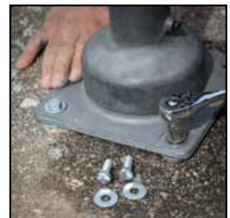
USING A 9/16" RATCHET, TIGHTEN BOLTS
