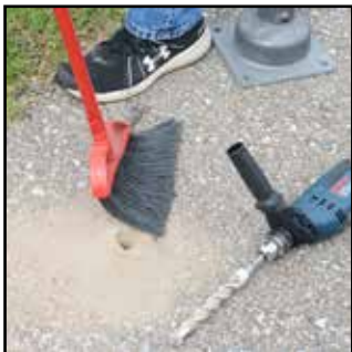
CLEAR AWAY ANY DUST OR DEBRIS
