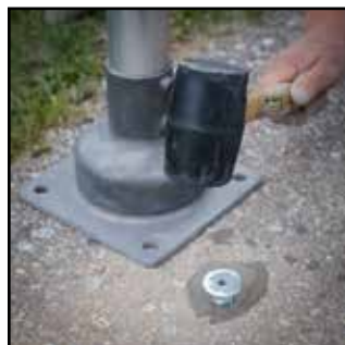
USING A RUBBER Mallet, TAP BOLTS INTO THE HOLES
