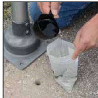
SLOWLY MIX APX. 3/8 CUP WATER WITH GROUT MIXTURE (DON'T DUMP ALL THE WATER, ADD JUST A LITTLE AT A TIME)
