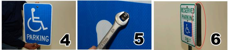
• Using your sign as reference, move the bottom mounting bracket into place and tighten the set screws, securing the brackets to the pole
