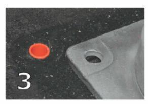
• Use a rubber mallet to tap the expansion plugs into the drilled holes
