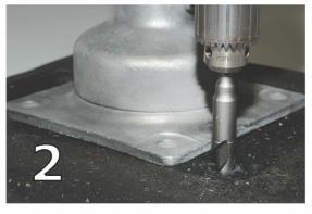
• Using a 3/4" masonry bit, drill 5" in depth
