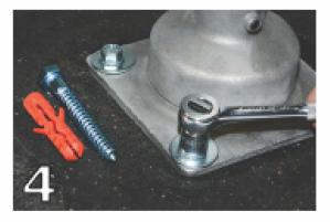
Place the base plate over the four holes and use a socket wrench with a 15/16" drive to thread all four hex lag screws into the expansion plugs
