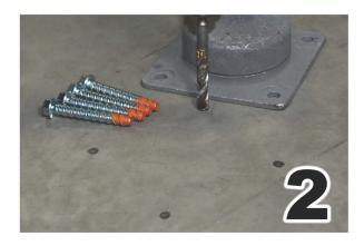
• Using a 1/2" masonry bit, drill 5" in depth
