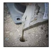
**POUR MIXTURE INTO THE 4 HOLES** (ONE BAG PER TWO HOLES)
