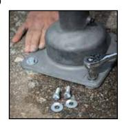
**USING A 9/16"** RATCHET, **TIGHTEN BOLTS**
