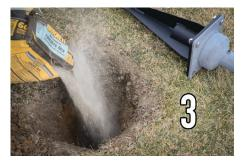
Remove base, fill hole with quick setting concrete.
