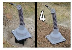
Place the XL Base and ground spike in the concrete. Fill the rest of the hole with excess dirt
