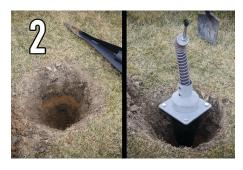
• Dig a hole apx. 18" deep and 6" wide. Put the ground spike in the hole to make sure the XL base is level with the ground
